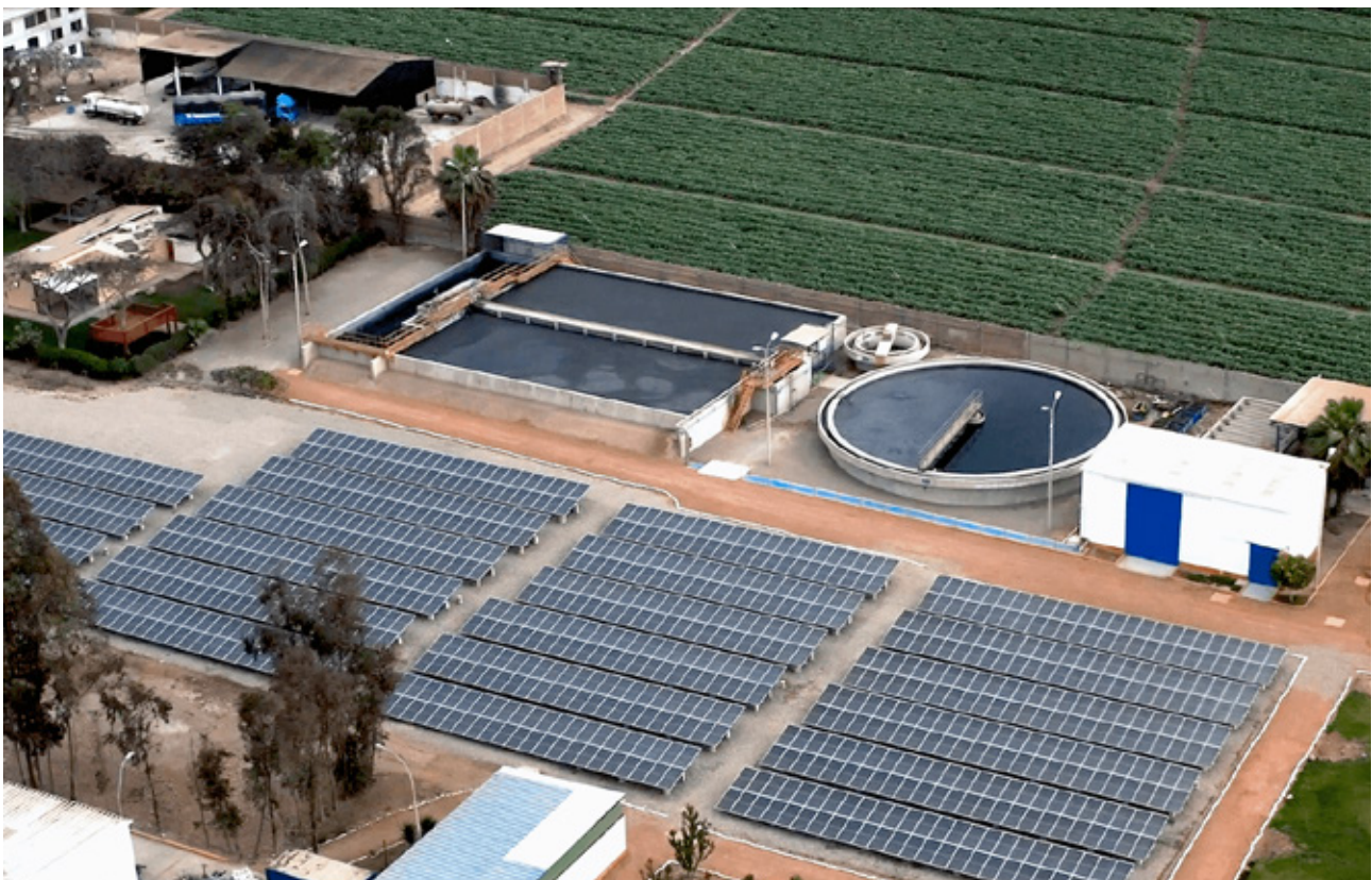
WWTP in Chincha Branch
